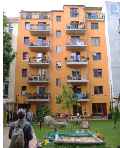
Low-energy Berlin apartment building – with wood pellet and solar-assisted heating system
